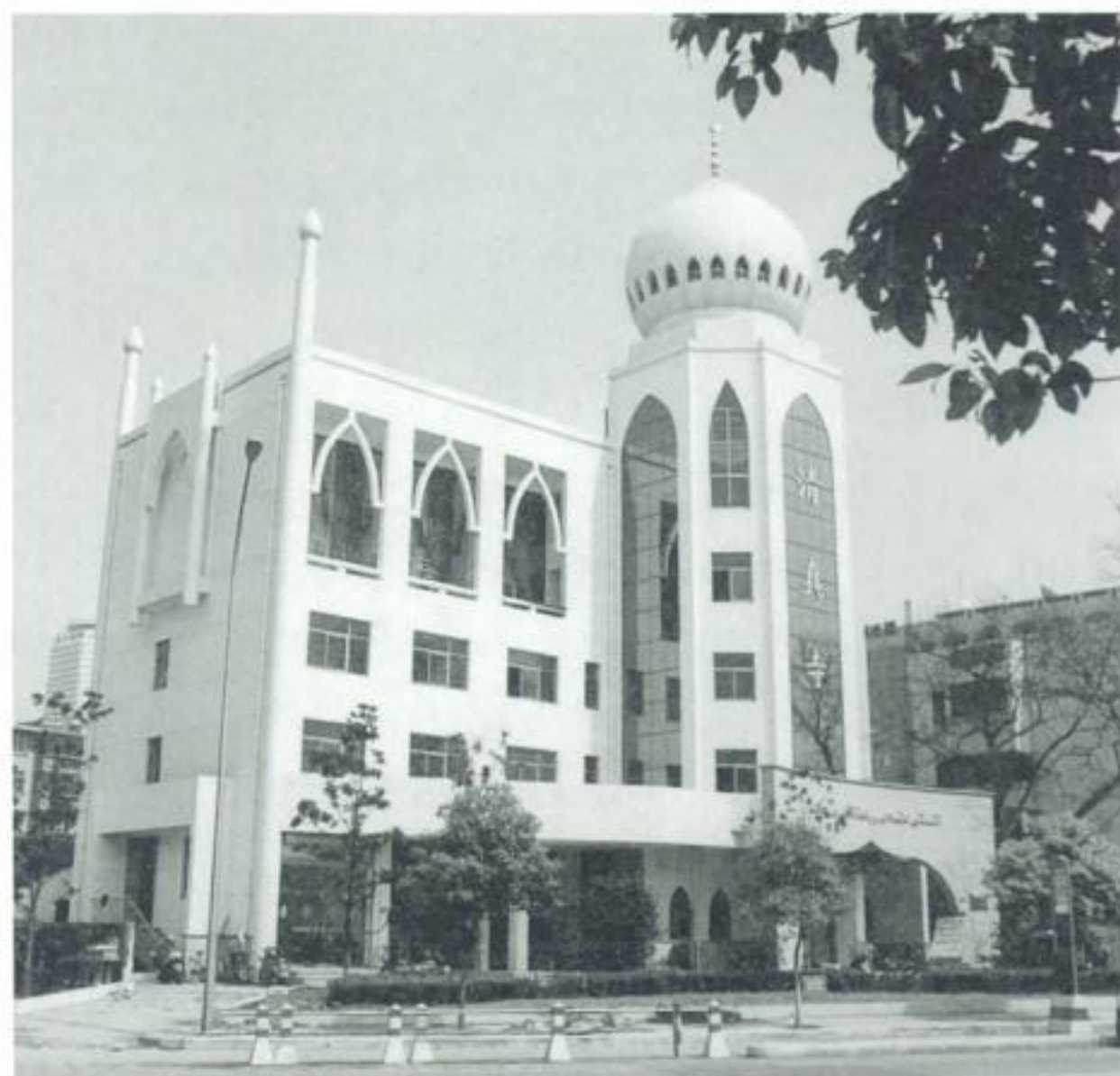
© New built Pudong Mosque in Shanghai.
